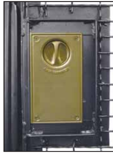
Standard back with recessed thumb turn.
